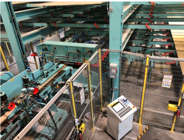
View of the lumber processing equipment
